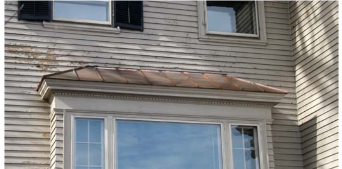
Left page: Steel erection for the library addition in November 2017. Right, from top: The finished roof on the Goddard-Daniels House; copper edging on the awnings.
