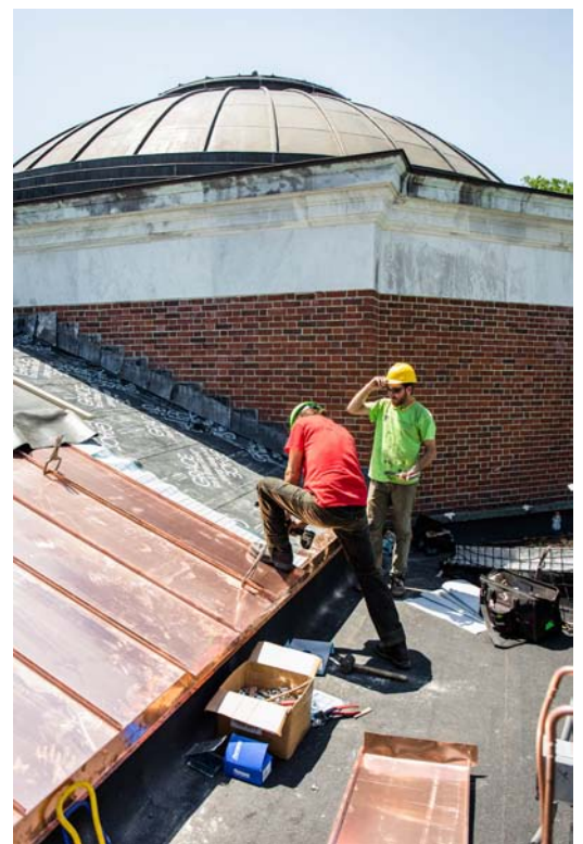
Above: Copper workers near the dome—exterior on the roof of Antiquarian Hall in startlingly similar photos taken by photographers over a century apart.
